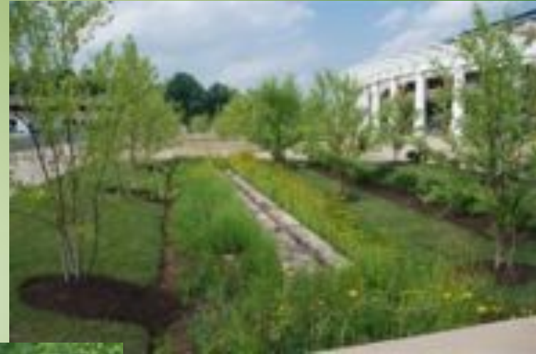
Innovative Stormwater Management at John Paul Jones Arena
