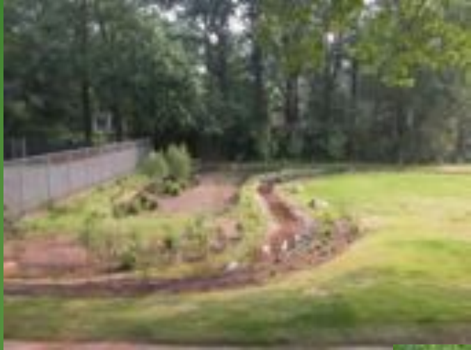
Stream Restoration at The Dell
