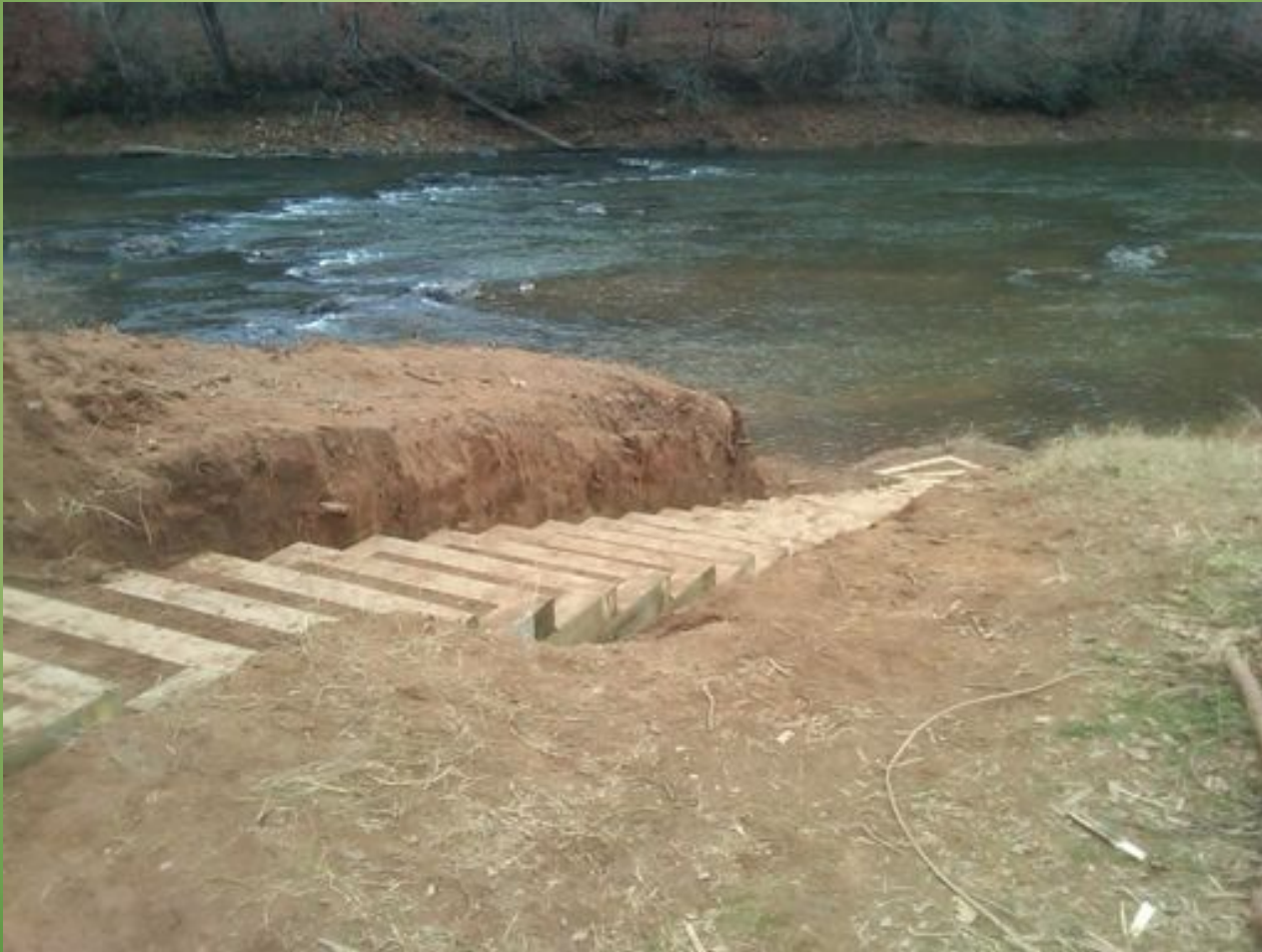
New staircase at Riverview Park – Eagle Scout project
