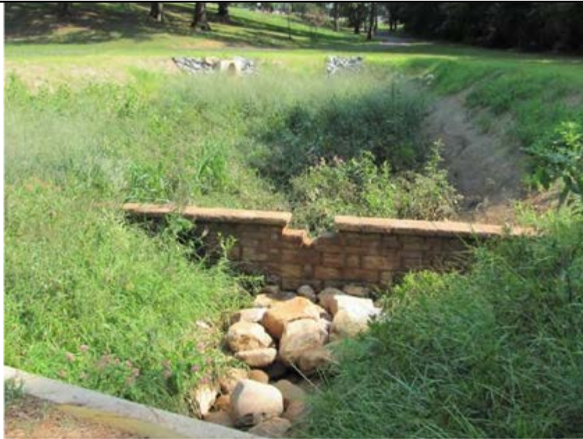
Forest Hills Park Daylighting and Water Quality Swale - After
