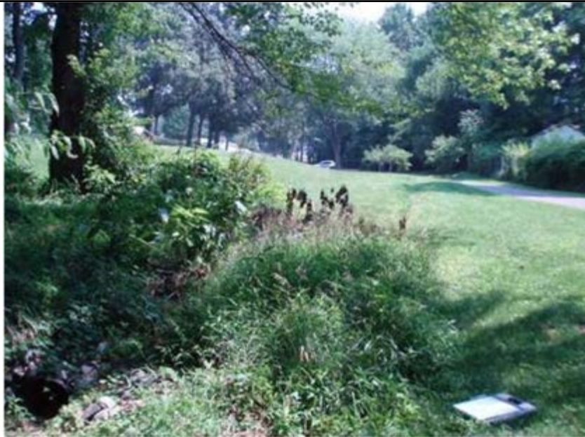
Forest Hills Park Daylighting and Water Quality Swale - Before
