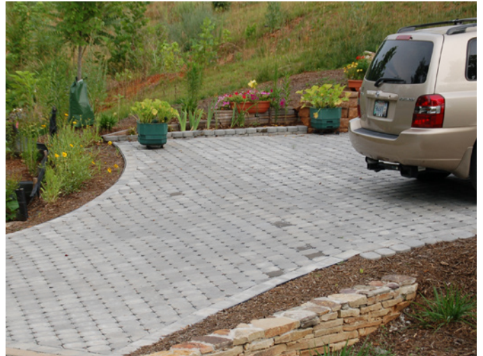
Porous pavers allow rainwater to percolate be absorbed into the ground below. A few recent projects in our area have incorporated them for parking areas and driveways, like the RiverBluff development in Charlottesville.
