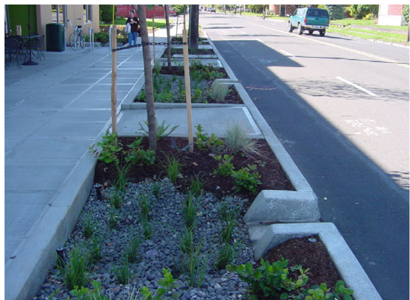
Periodic curb cuts allow some street runoff to drain into planting areas like the ones pictured in the example above.
