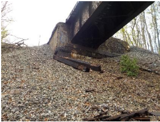
Figure 7: Wooden ties under Railroad bridge
