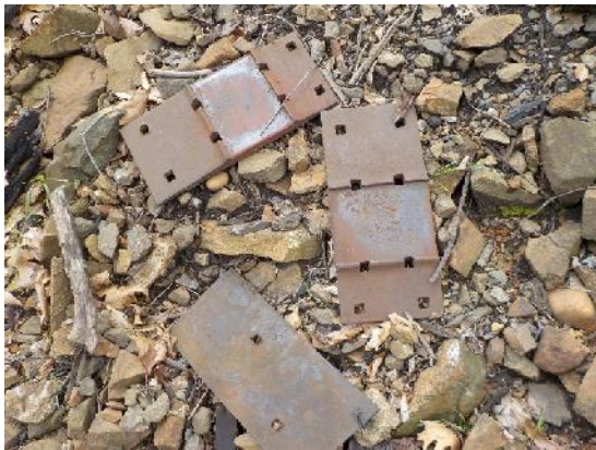
Figure 5: Steel tie plates under Railroad bridge
