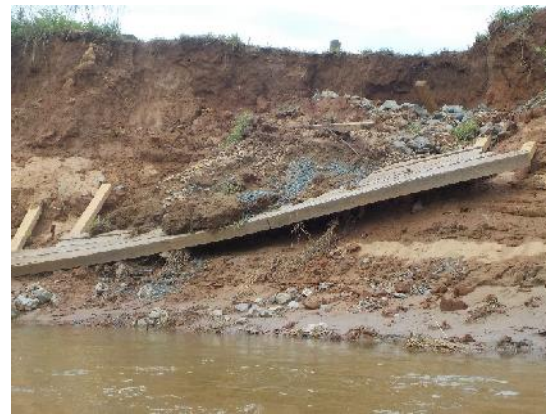
Figure 16: Wooden wall washed out at Glenmore trail
