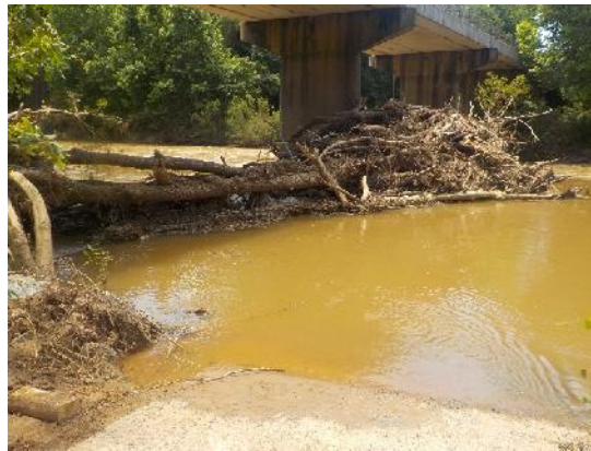
Figure 4: Tree debris blocking River at Crofton Bridge
