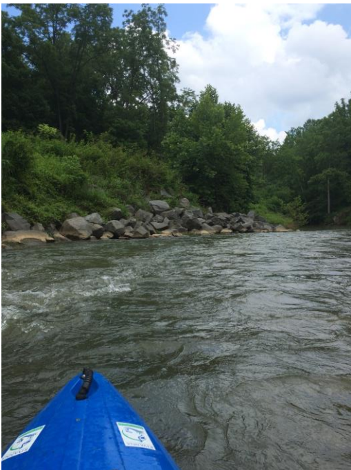
Figure 7: Manmade rock riprap near dam.
