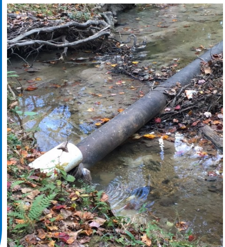
Lake Monticello broken sewer pipe in stream
