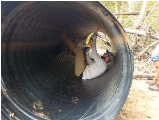
Figure 9: Mario sawing the pipe into pieces
