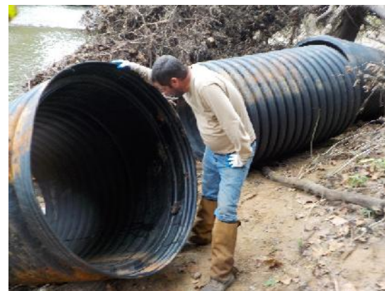
Figure 11: Removing water from pipes to make them lighter
